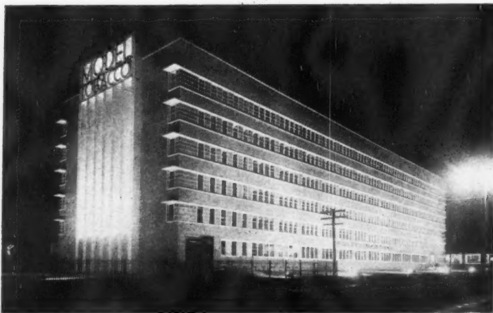
Floodlights give "that added touch" to the attractive Model Tobacco plant of the United States Tobacco Company in Richmond. Credited with being the outstanding industrial building in the South, this plant is modern to the last detail and may be considered representative of the well-planned "industrial building of tomorrow." G-E floodlights illuminate both sides of the buildings and the pilasters at each end.
